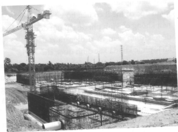
Thu Duc, Ho Chi Minh City Build own Operate (B.O.O) under construction May 2006
